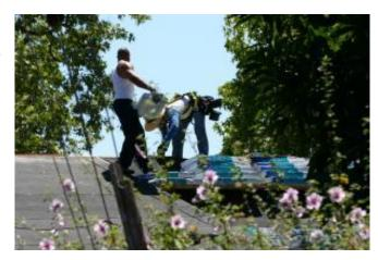
5. Wear some type of safety harness while working on high, unprotected surfaces, like a ROOF!
